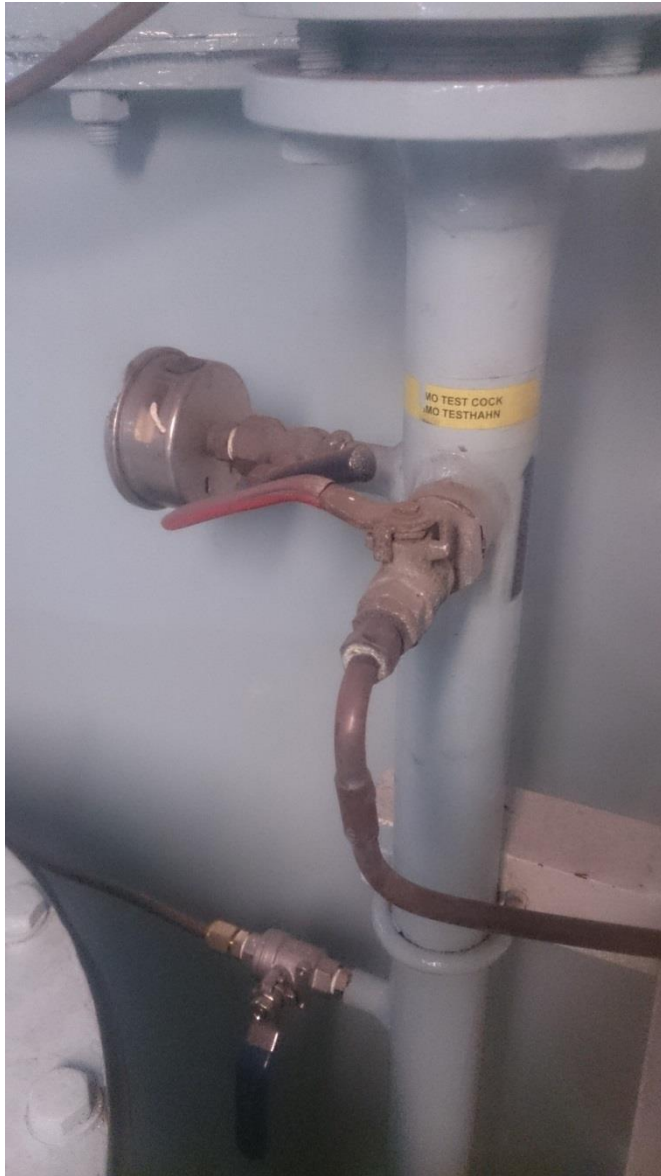
Fresh water connected to overboard line before Oil Content Meter
