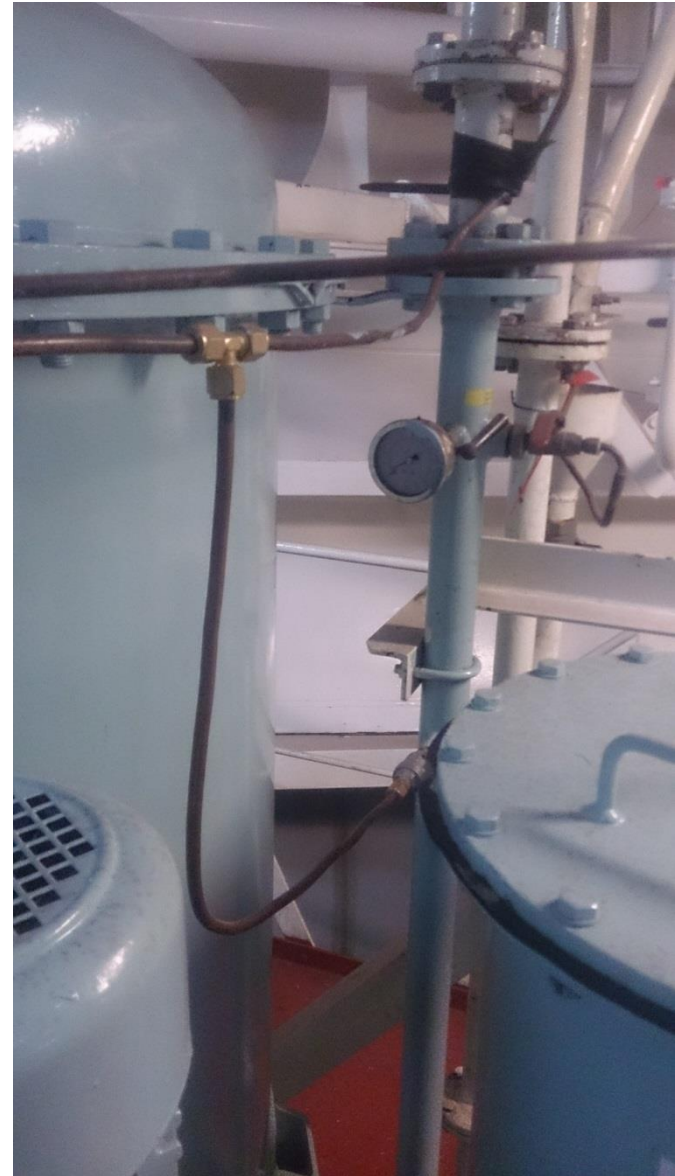
Fresh water connected to overboard line before Oil Content Meter
