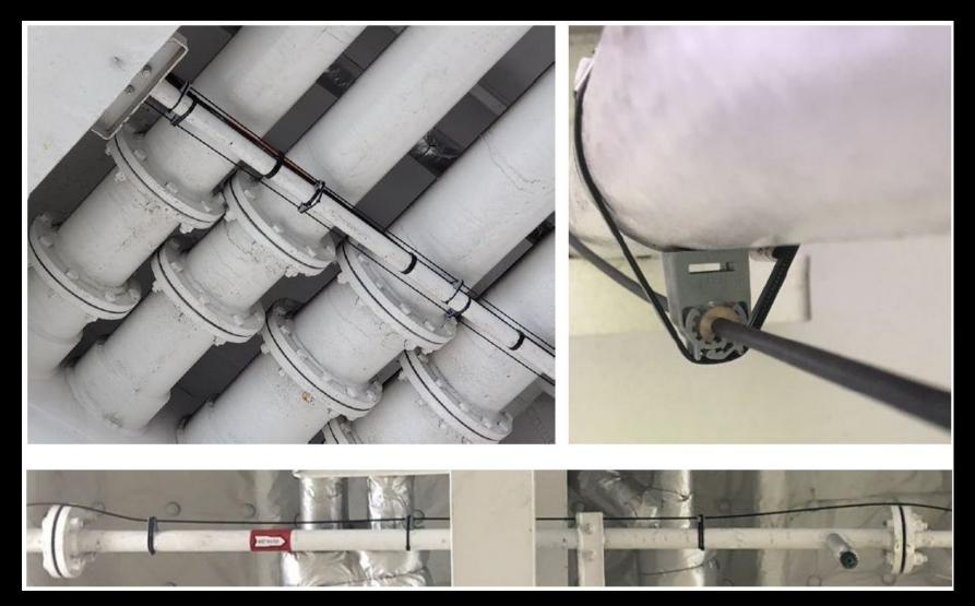
A single fibre-optic cable can be used to monitor temperatures along the deckhead up to a distance of 16 km.
